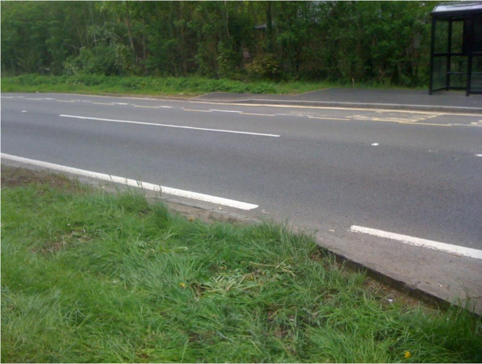
Close-up of the verge where the path would need to be sited (approximately)
